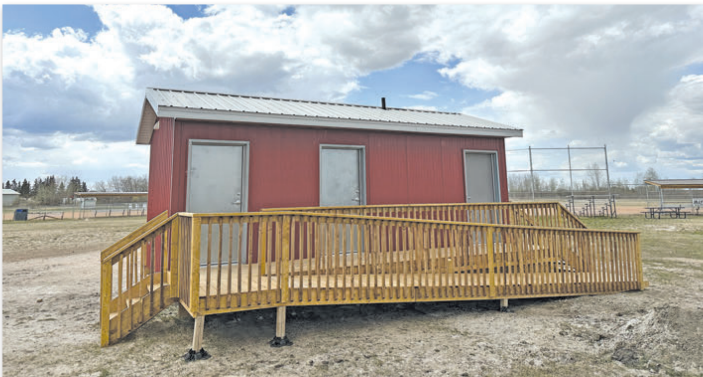
Thanks to the work of Spiritwood's Ball Diamond Restoration Committee, the ball diamonds at SADSAC park now have a washroom facility with running water.
