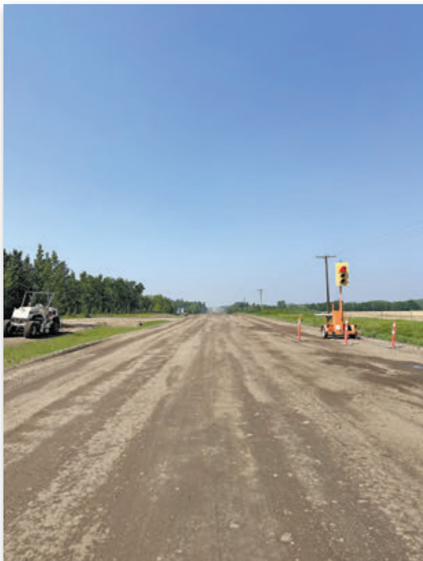
Construction is underway on Highway 24 between Leoville and Chitek Lake.
