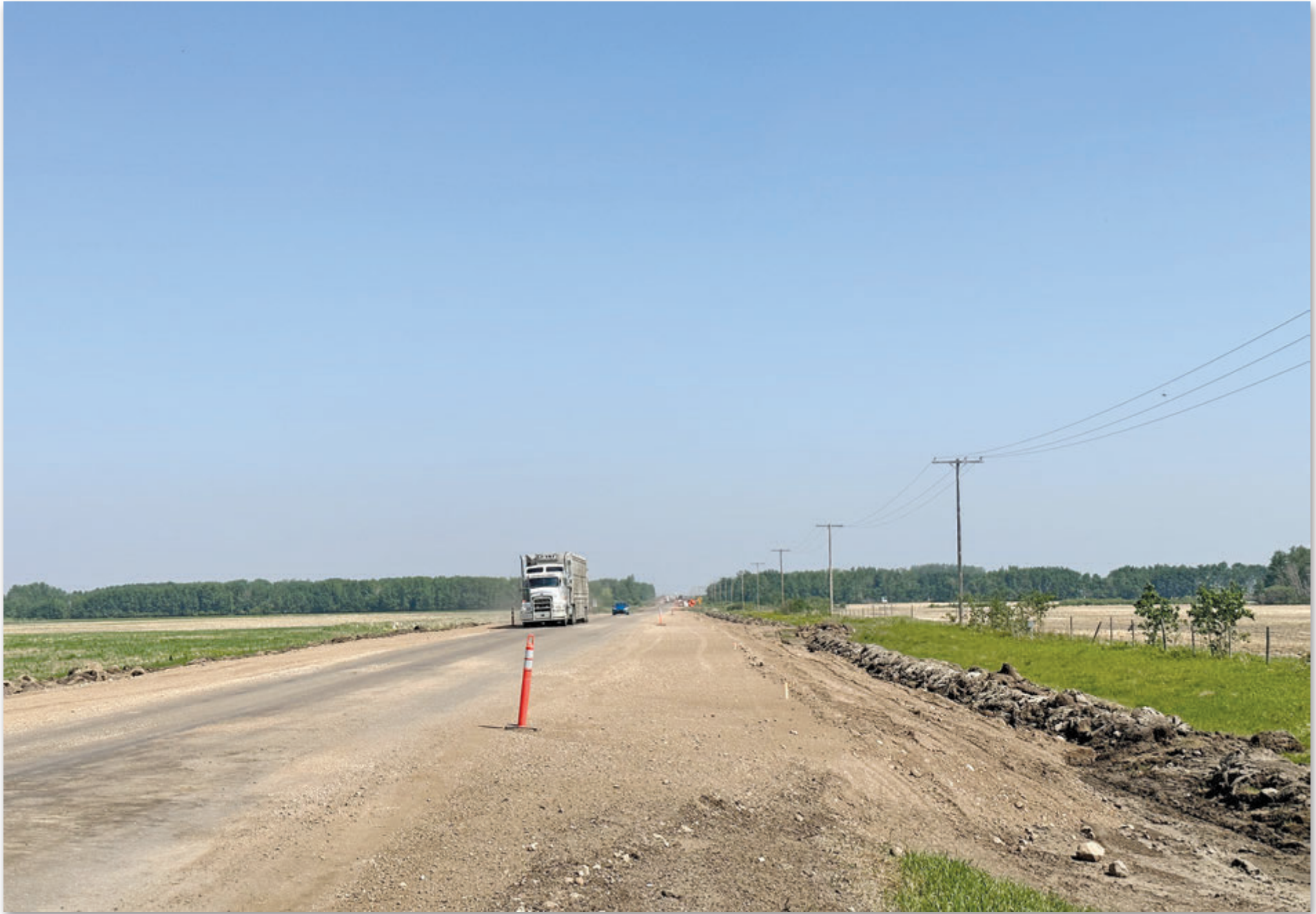
Construction is underway on Highway 24 between Spiritwood and Leoville.
