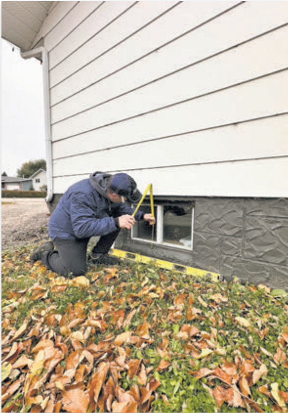
Committee volunteer Bryan Wingerter gleans the window measurements for the checklist of renovation items.
